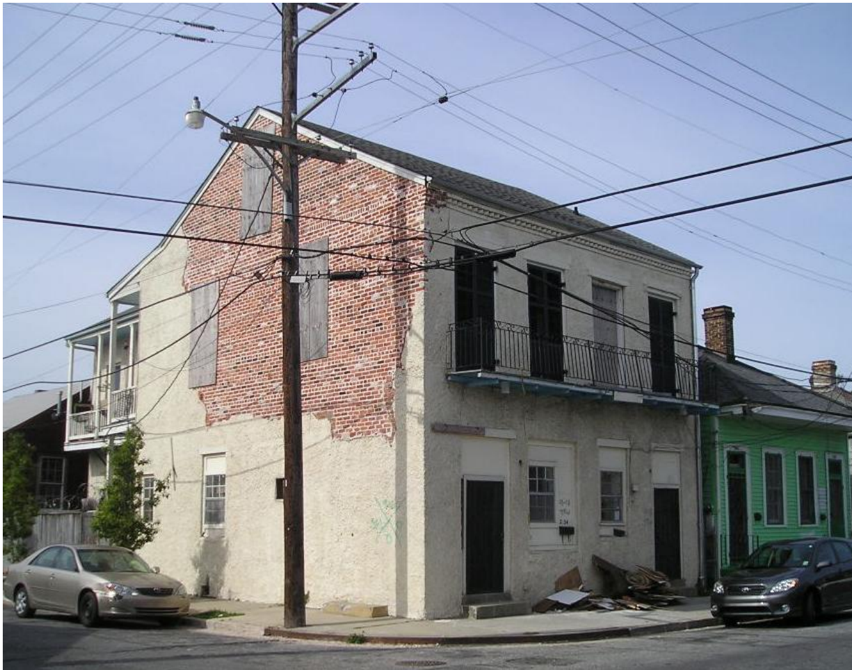
March 26, 2007 – Evidence of beginning of building stucco finish delamination cited by HDLC.
