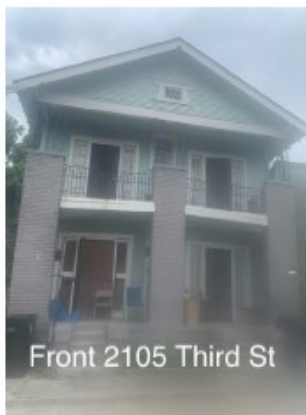
Photo submitted with Demolition application, 2025
