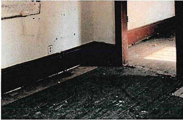
Floor is sinking – piers are sinking
