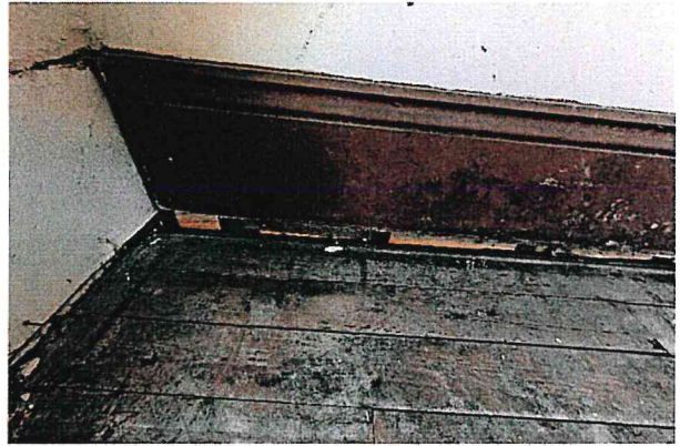
Floor is sinking – piers are sinking
