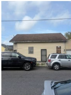
Photo submitted with Demolition application, 2025
