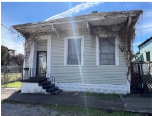
Photo submitted with Demolition application, 2025
