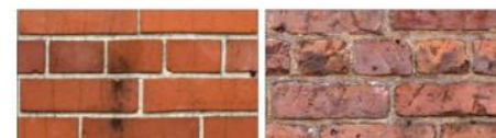
20th Century Brick – A hard, dense, fired-clay, regularly shaped building component; sometimes with a glazed surface; used primarily in walls, piers, foundations and exterior pavers.
