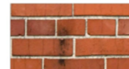
20th Century Brick – A hard, dense, fired-clay, regularly shaped building component; sometimes with a glazed surface; used primarily in walls, piers, foundations and exterior pavers.
