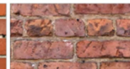
19th Century Brick – A soft, fired-clay, fairly regularly shaped building component; often with color and surface variations; used primarily in walls, piers, foundations and exterior pavers.
