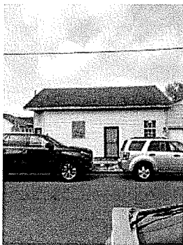
Photo submitted with Demolition application, 2025
