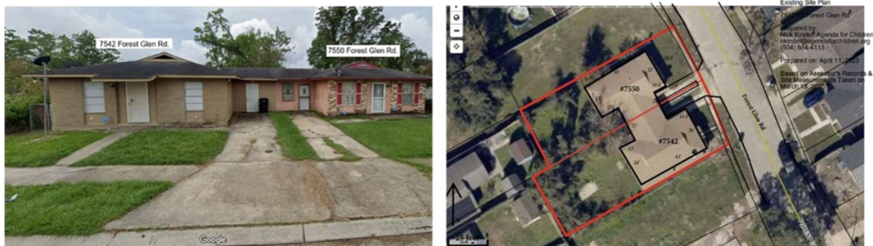
Figure 1. Front and Aerial View of the Structure
