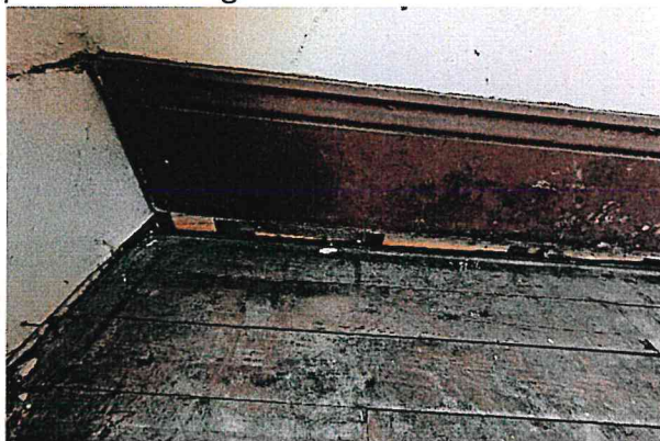
Floor is sinking – piers are sinking
