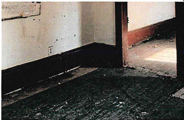
Floor is sinking – piers are sinking
